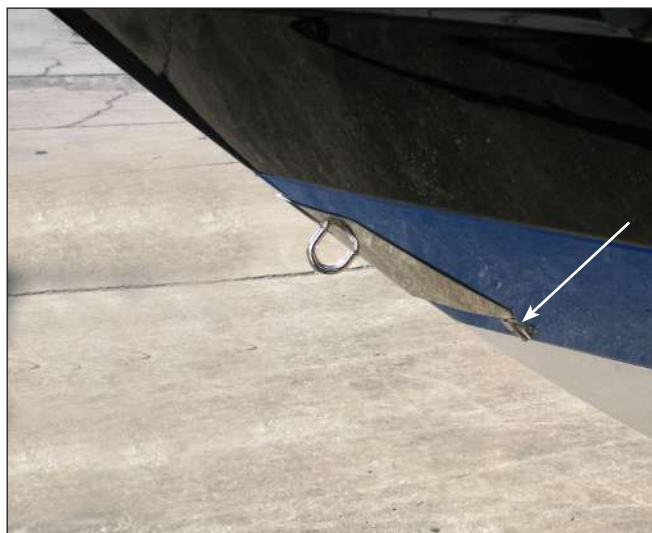
Rope Locker Drain
