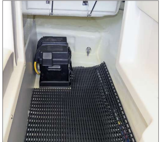
Battery Location In Storage Compartment
